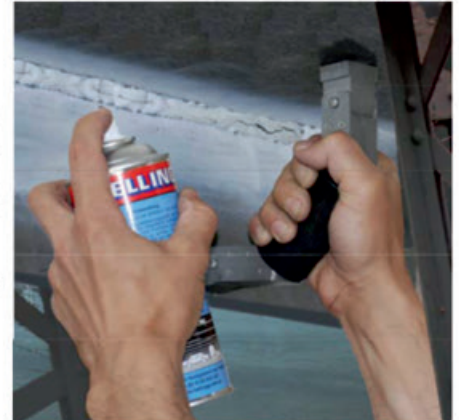
Weld joint inspection on a bridge by use of BW 333 black magnetic particle suspension and NR 104 A white background paint.
